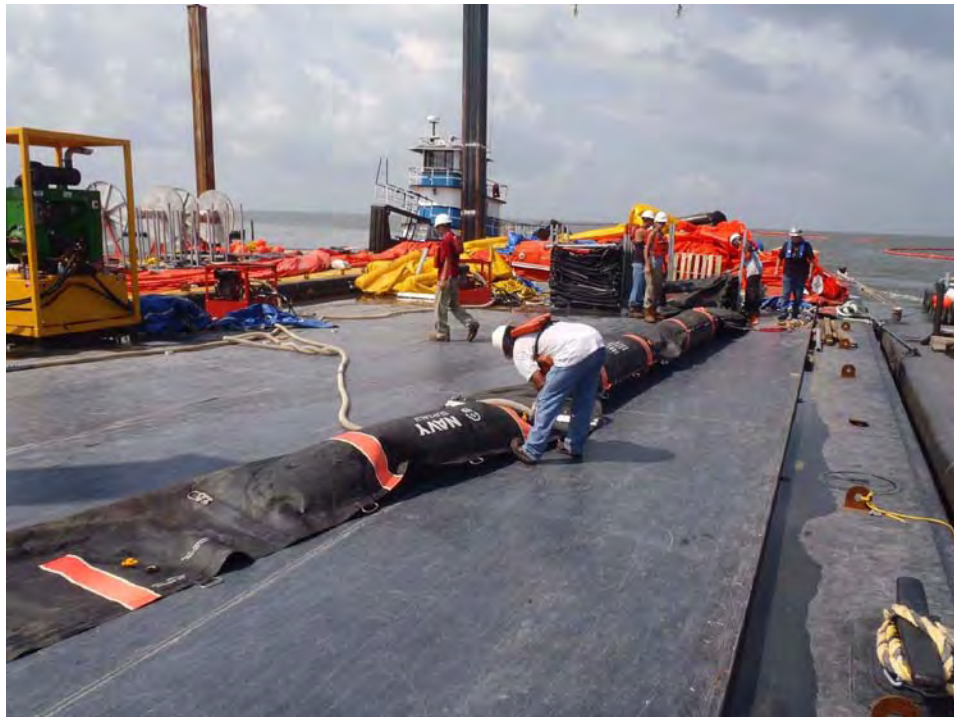
Figure 5-15. June 6 2010 image of crews on OSV WES BORVELON preparing boom for deployment in vicinity of Half Moon Island, LA where pilings were driven as boom attachment points.
