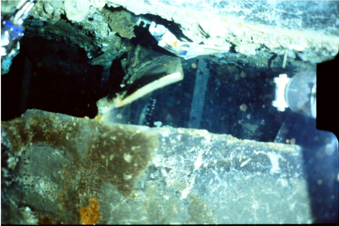
Photograph 13: Pontoon Leg Separation from the Main Platform Box
