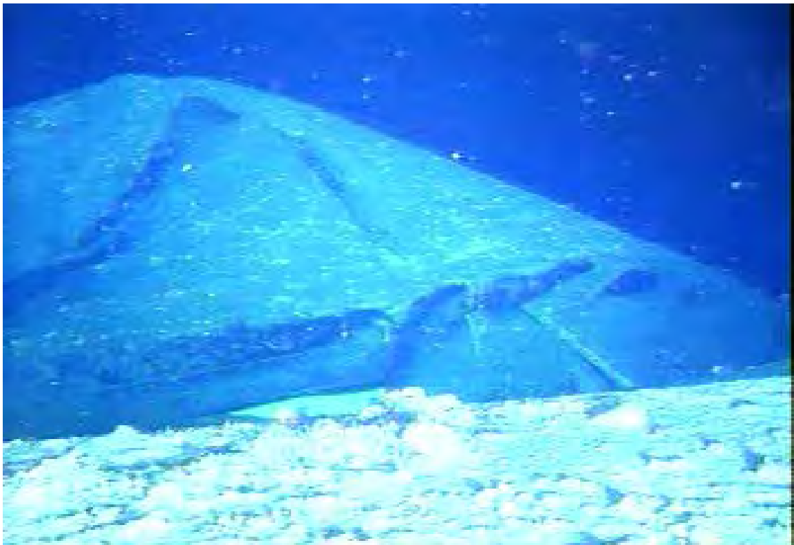
Photograph 10: Deep Water Horizon Pontoon Damage Port Side
