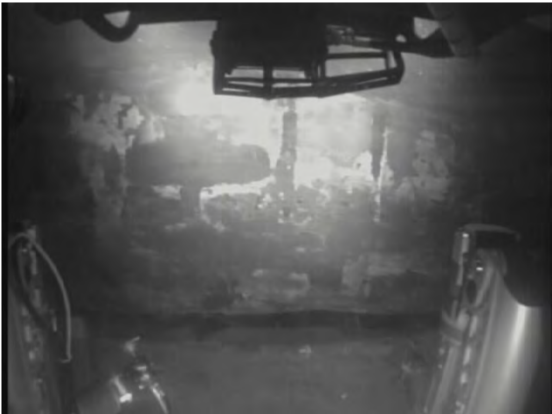
Photograph 12: Pontoon Leg Separation from the Main Platform Box
